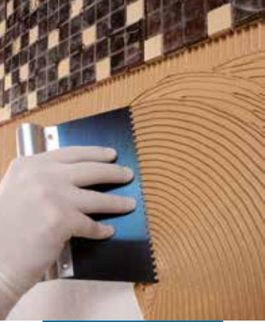
Spreading the adhesive with a Mapei No. 4 trowel
