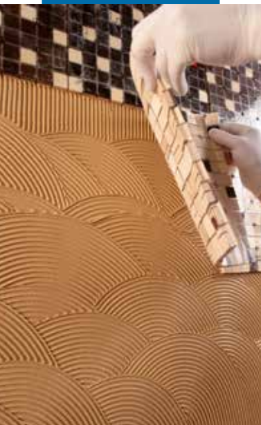
Applying the sheet of mosaic
