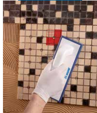
Pressing the mosaic down well and adjusting it into the correct position
